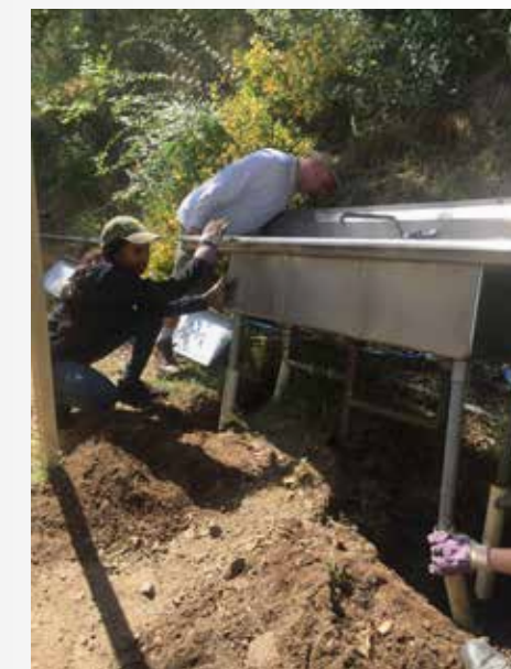
Rockwell Automation installing wash basin at Big Oak Canyon
